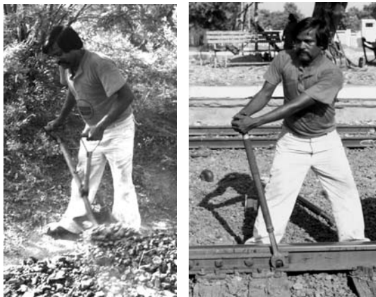
Figures 8 & 9 Gang men are working with the newly developed prototypes of shovel and spanner
